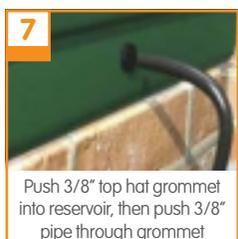
Push 3/8" top hat grommet into reservoir, then push 3/8" pipe through grommet
