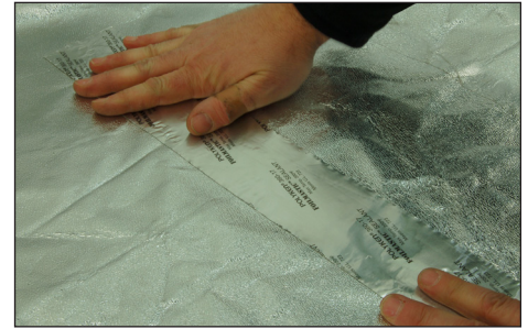
STEP 3: Firmly press the tape over top of the tear to bond the skin back together.
